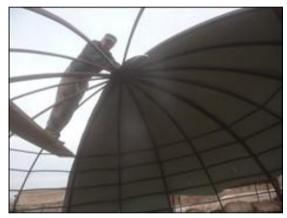
The dome was covered with the metal sheets, and the gaps between the sheets were filled with silicon to maximize the protection.
