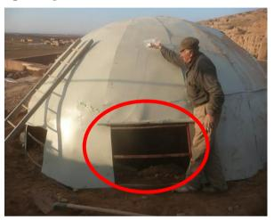
The next stage was in 2014, when we turned our attention to the Abi entrance. The entrance was then also covered with a metal grid that was fixed and welded, then covered with overlapping metal sheets.
